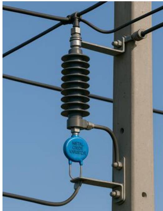
Gambar 2. Aresster Tipe Metal Oxide Varistor MOV
